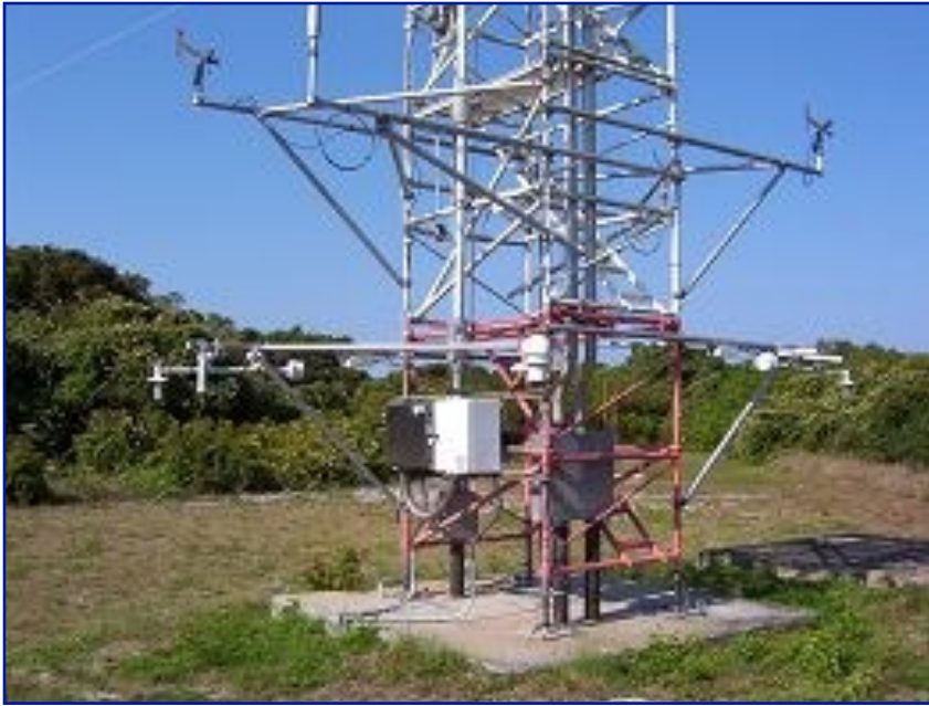
Figure 10. Photograph of tower 6 showing redundant wind sensors at a height of 12 ft on opposite sides of the tower.
