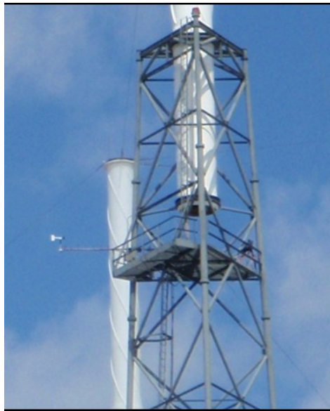
Figure 4. The SLC 41 southeast lightning protection tower and wind sensor, looking west-northwest. The top of the southwest lightning tower is in the background.
