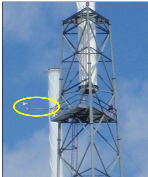
Figure 18. The SLC 41 southeast lightning protection tower and wind sensor, looking west-northwest. The sensor and boom are highlighted by the yellow ellipse. The top of the southwest lightning tower is in the background.
